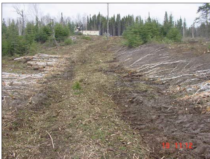
Brush mat used to cross wetland.
