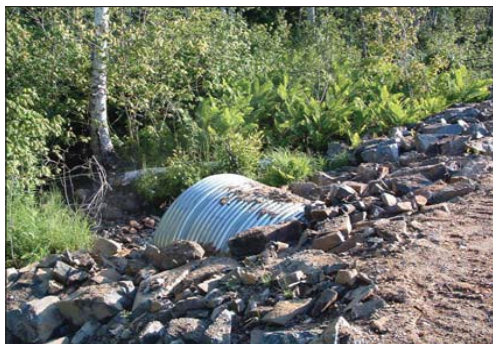
Proper use of rock for sedimentation control.
