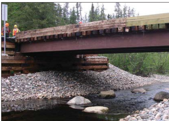
Proper sediment control on bridge structure.
