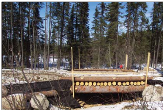
Geotextile used to prevent stream siltation.
